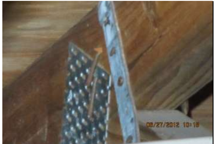
Roof-to-Wall Connection Single Wrap, 4 Nails, Opposing Side
