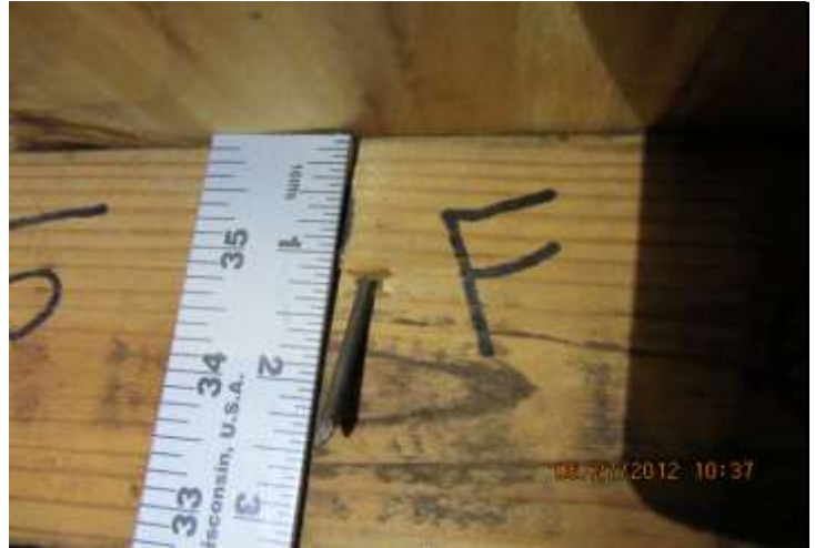
Roof Deck Attachment 8d or Larger Nail
