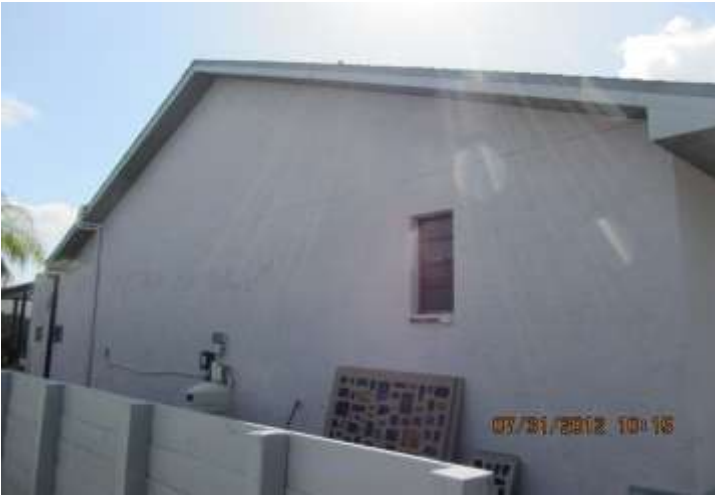
Left Elevation Unprotected, Unrated Glazed Opening
