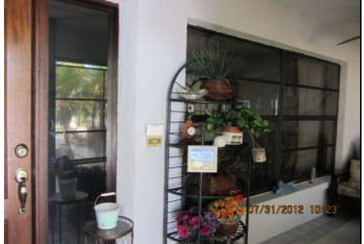
Opening Protection Unprotected, Unrated Glazed Openings
