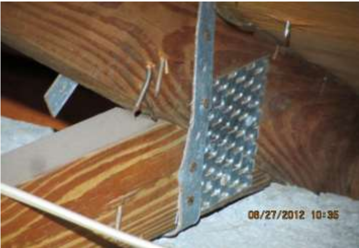
Roof-to-Wall Connection Single Wrap, 4 Nails, Anchor Side
