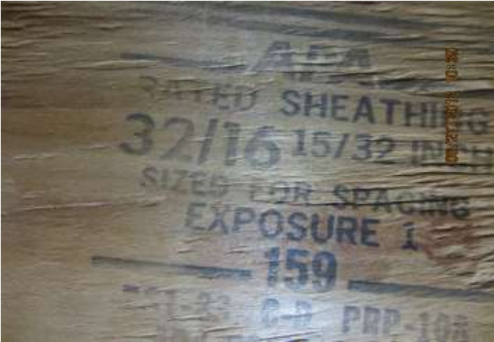
Roof Deck Attachment 15/32 Thick Plywood Roof Deck
