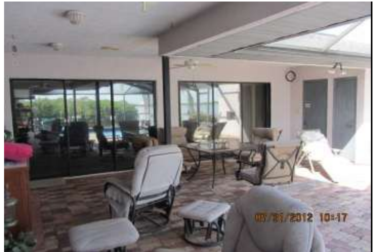
Opening Protection Unprotected, Unrated Glazed Openings
